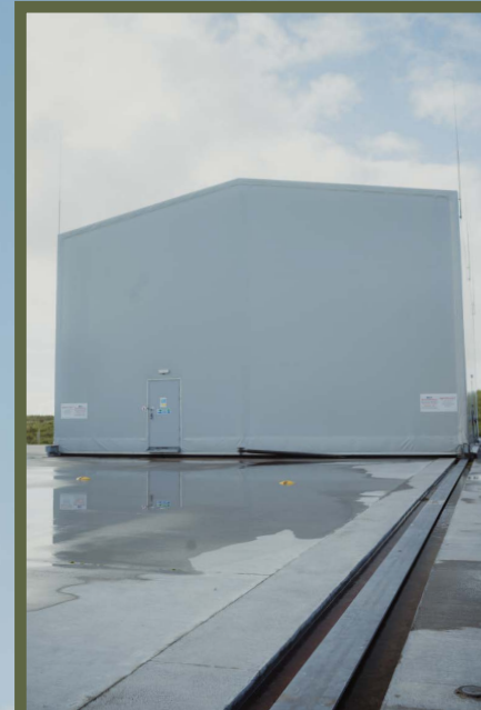
The building will pull back along these rails to reveal the asset.
